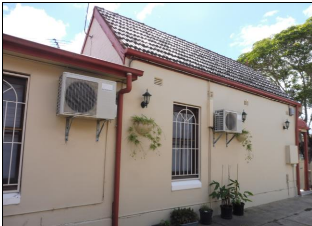
Figure 5.6 The front wing retains the main gabled roof form and one window opening on the southern façade.
