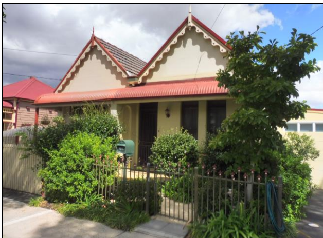
Figure 4.4 No. 53 also retains the openings and matching details on the front façade. A solid party wall separates the two front verandahs which have a continuous bullnosed hipped roof.
