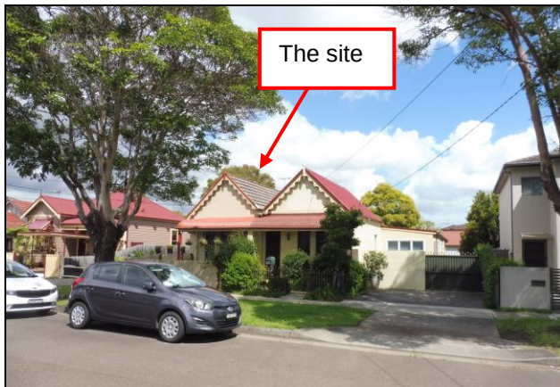
Figure 4.2 The subject building is part of a pair of Victorian semi-detached dwellings that with No. 53 retains the main gabled roof form with gables facing the street.
