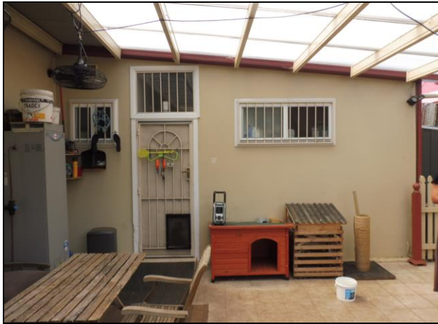
Figure 5.9 The existing rear wall and rear verandah.
