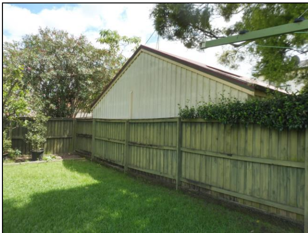
Figure 5.14 A large gable roof structure at the rear of No. 53 is constructed to the shared boundary.
