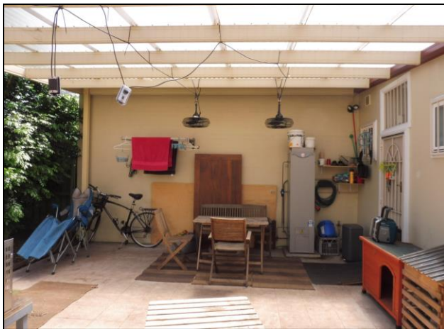
Figure 5.10 The rear verandah has a modern tiled floor and skillion roof and is also bounded by the shared boundary/ party wall with No. 53.
