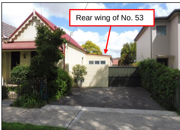
Figure 4.5 The deep setback, hardstand fence and gate in the northern setback of No. 53. The rear wing of No. 53 has been extended to the rear and into to the northern setback.
