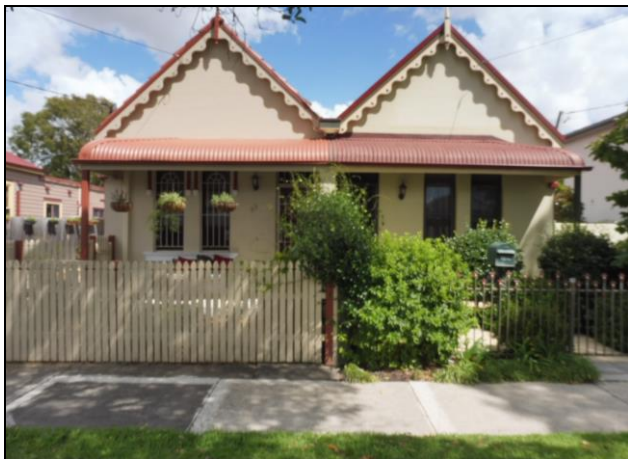
Figure 5.3 The front, Windsor Avenue façade which retains the street facing gable, pattern of openings, an open verandah and associated details that match No. 53 (at right).
