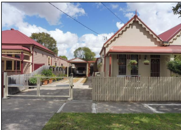
Figure 5.4 The building is sited close to but setback from the street frontage and has a deep setback from the southern boundary.
