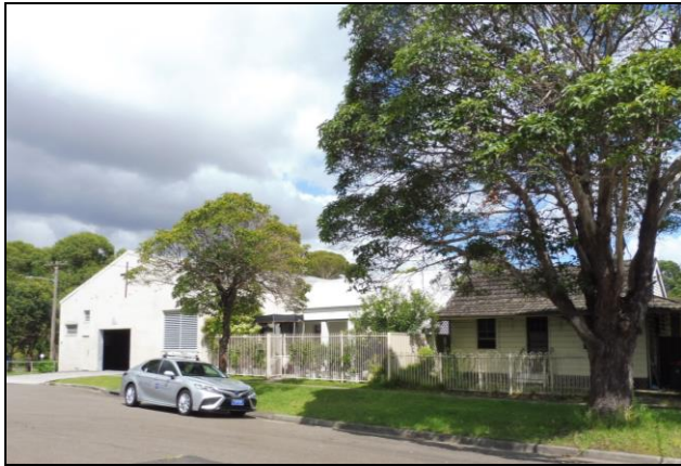
Figure 4.18 No. 65 and large hall/ Church building at the south western end of the street.
