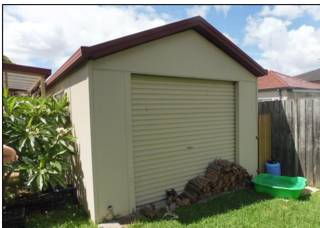
Figure 5.12 The existing garage is a lightweight structure with gabled roof and roller doors at each end.
