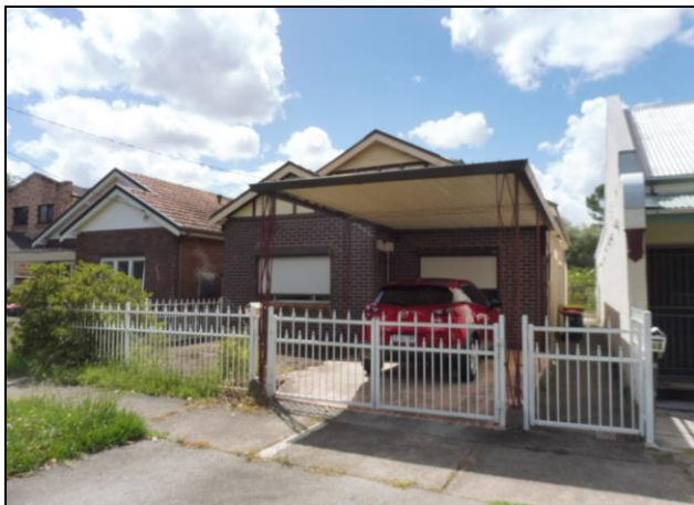
Figure 4.8 No. 58 Windsor Avenue.
