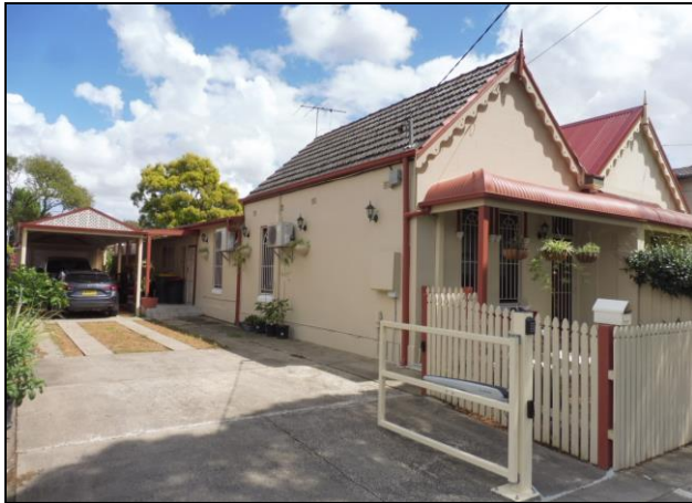
Figure 5.5 The southern façade and setback. A driveway and path extends along the southern side of the dwelling.
