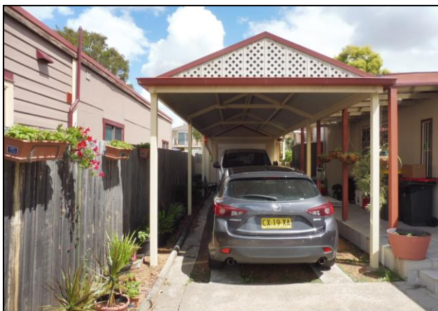
Figure 5.8 A steel framed carport and garage have been added to the deep setback adjacent to the rear wing.
